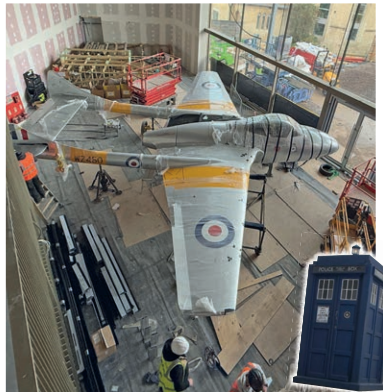
ICONS: Engineers install Vampire at Vanguard's Bath site. The firm also has displays of Doctor Who 's Tardis (inset), Spitfire and WWI Mark IV tank at its other premises
